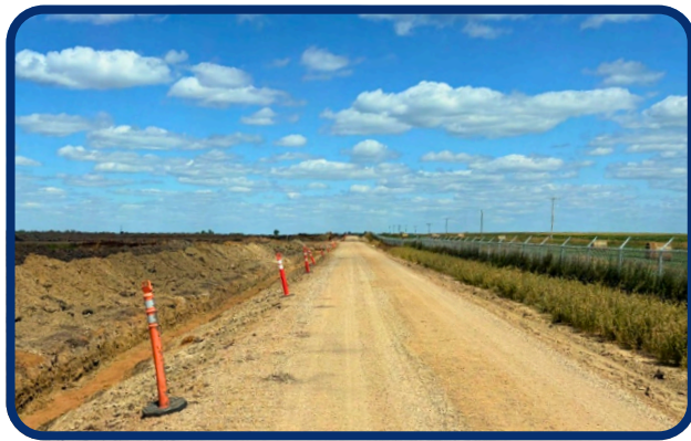
Representative Access Roads
