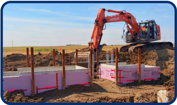
Representative Inverter Foundation
